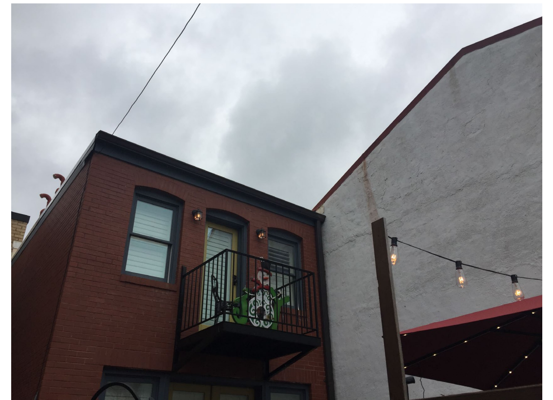
REAR FAÇADE @ 649 A STREET SE
