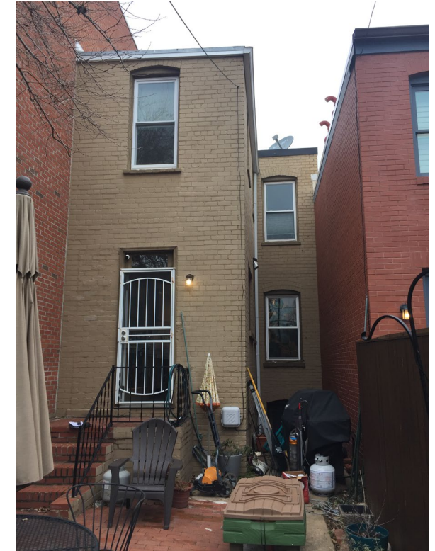
EXISTING REAR FACADE
