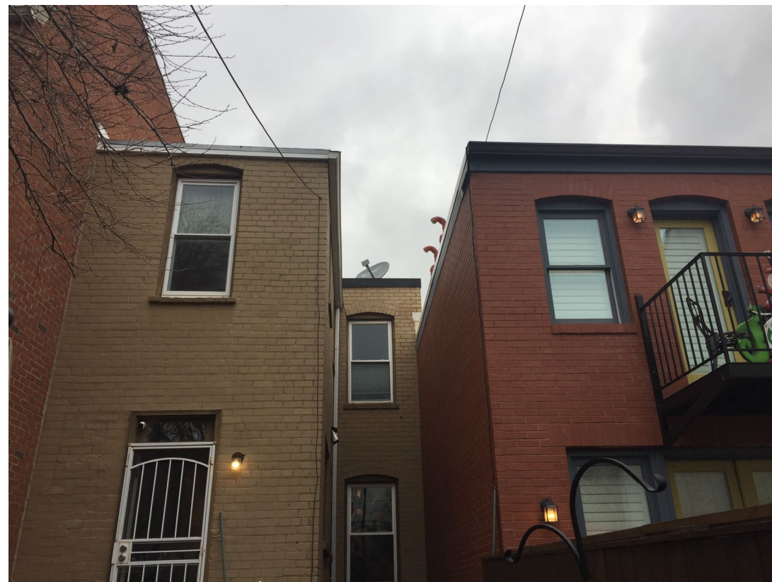
REAR FAÇADE, LOOKING EAST
