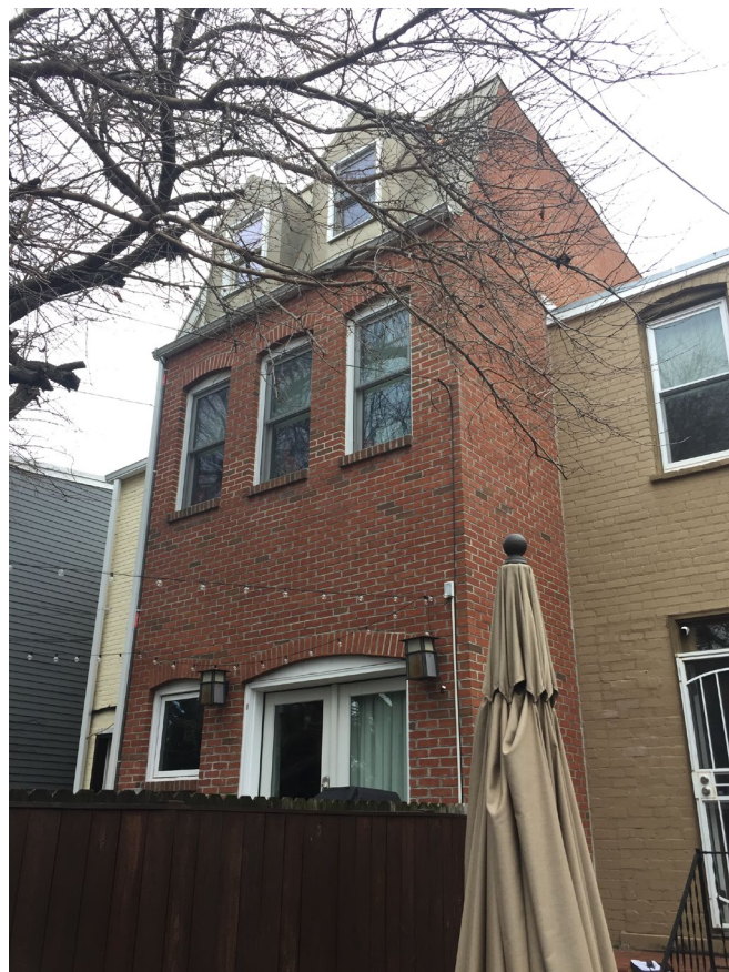
REAR FAÇADE, LOOKING WEST
